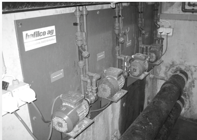
Messwasserpumpe
